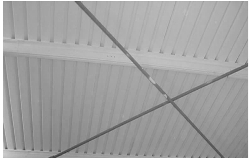
Steel roofing sheets in other premises
