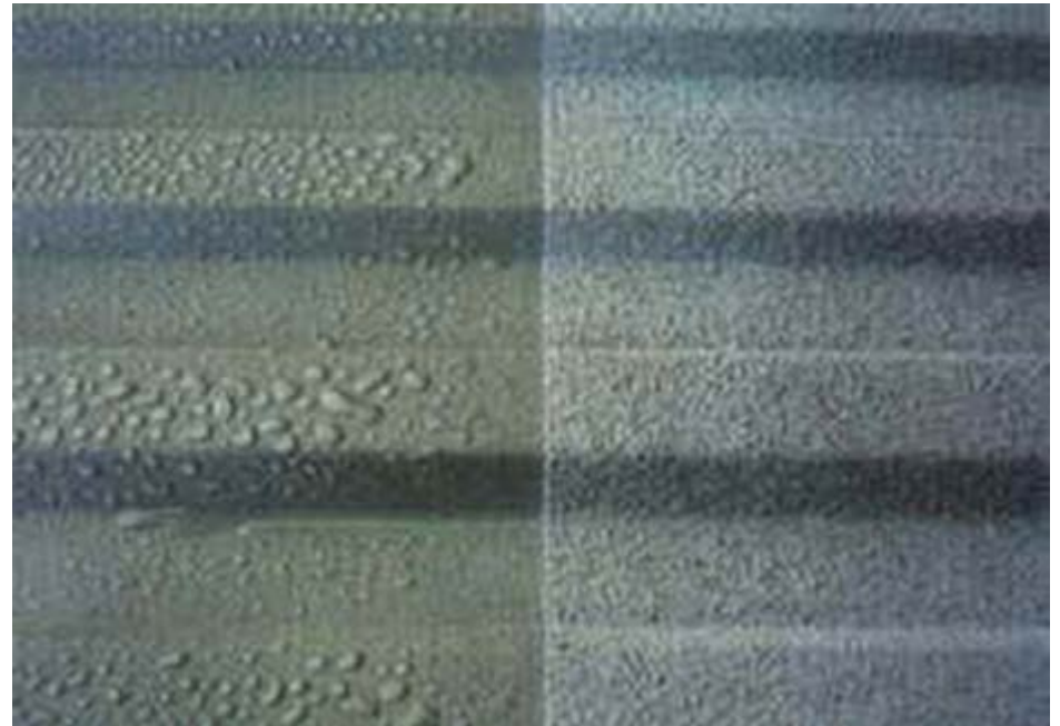
Untreated and treated with GrafoTherm steel roofing sheet
