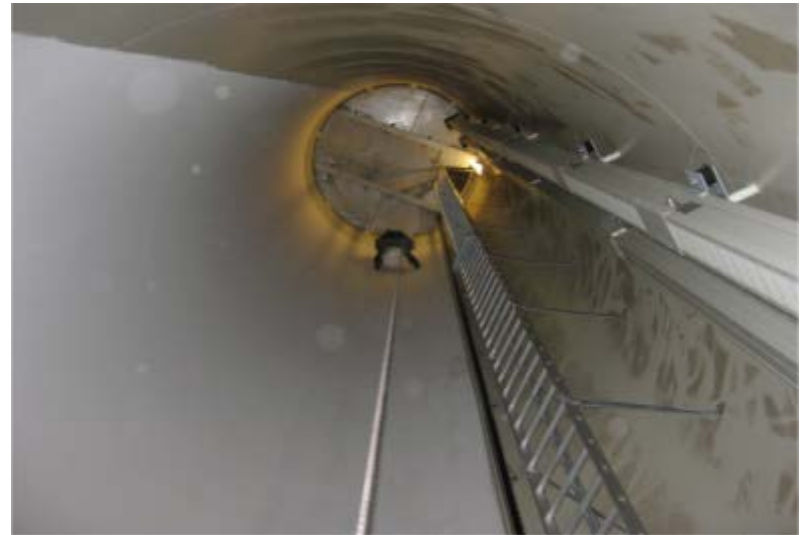
Interior surfaces of wind turbine towers
