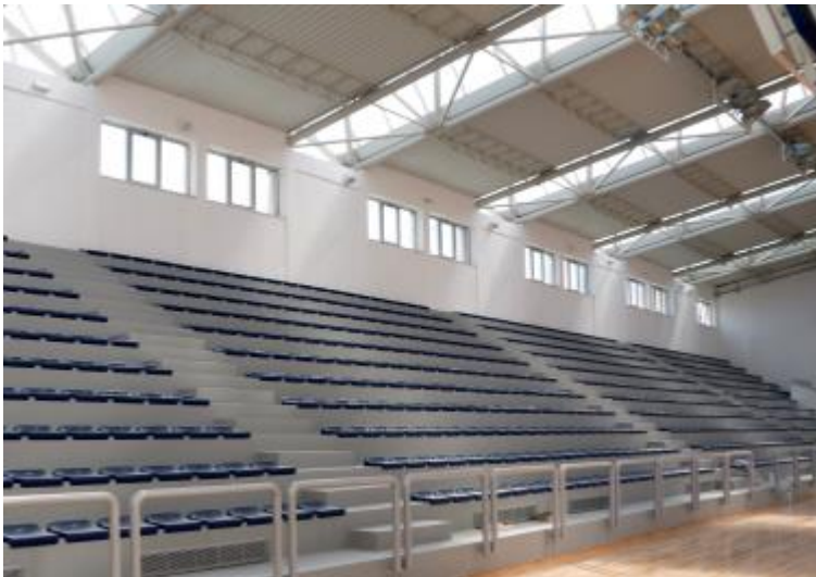
Steel roofing sheets and walls in sport facilities
