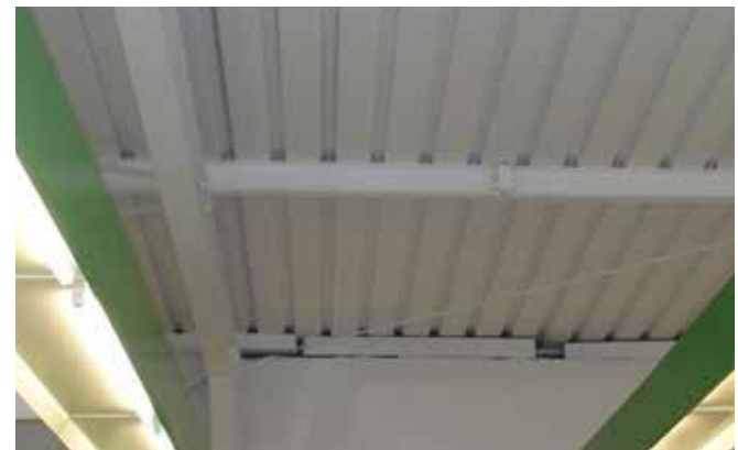
GrafoTherm anti-condensation coating on a roof plate
