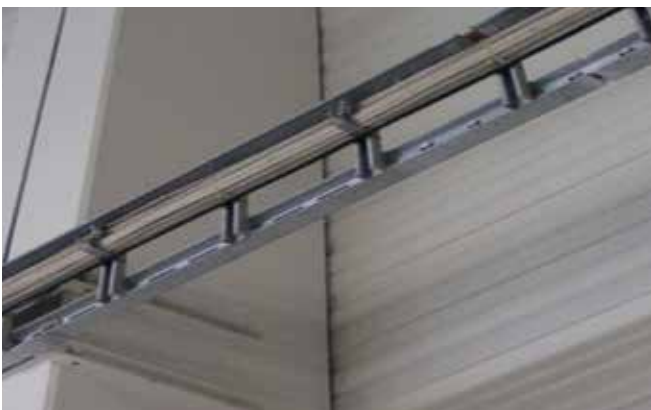
Sandwich boards treated with BioRid in a warehouse building
