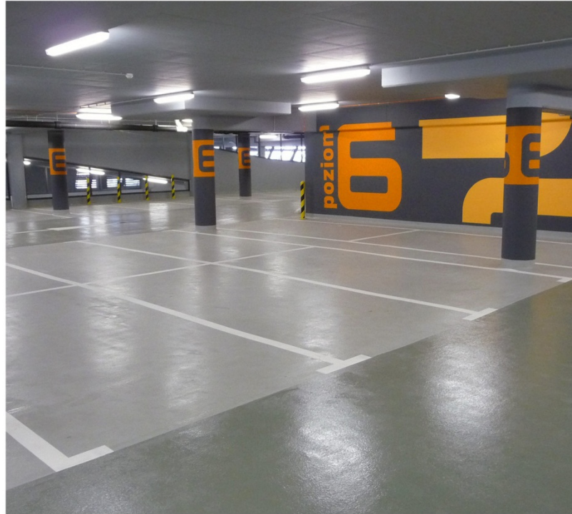
INDUSTRIAL SPECIFICATION Floors
